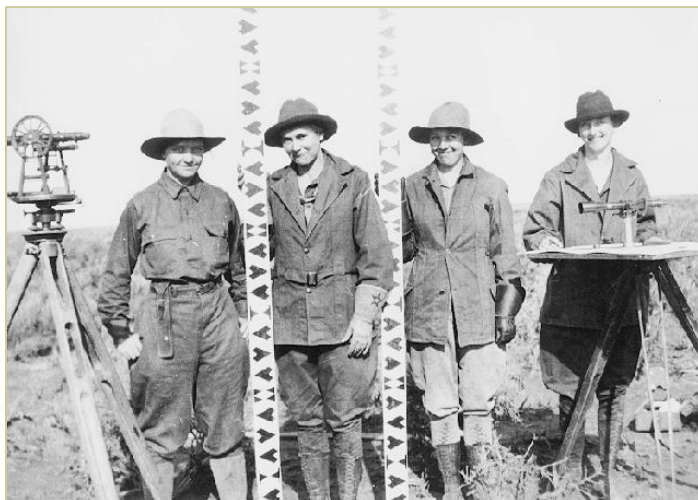
All female survey crew - Minidoka Project, Idaho 1918. Photo from the U.S. Bureau of Reclamation, of the U.S. Department of the Interior.
