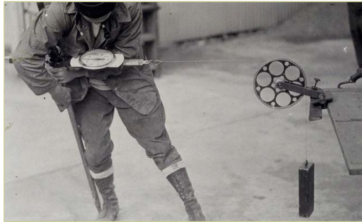
Steel tape with tape stretcher. Photo courtesy of National Oceanic and Atmospheric Administration, U.S. Department of Commerce.
