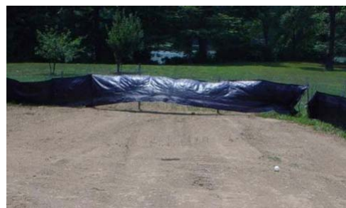
Silt fence must be trenched into the ground
